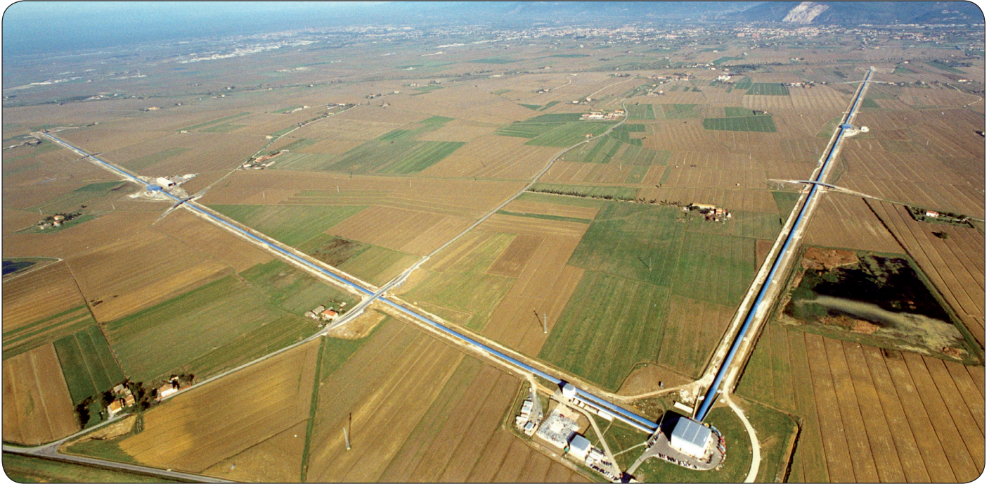
Fig. 5. The Virgo interferometer near Pisa, Italy. Both arms of the interferometer, each with a length of 3 km, can be seen.
