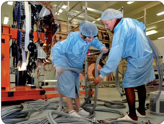
Fig. 2. Nikhef PhD students working on the SCT installation at CERN.
