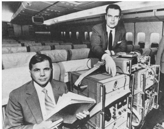
Figure 3.4: Atomic clocks were synchronized and taken on board of planes flying eastward and westward around the earth. After arrival they were compared and the prediction of relativity was seen to be correct.
