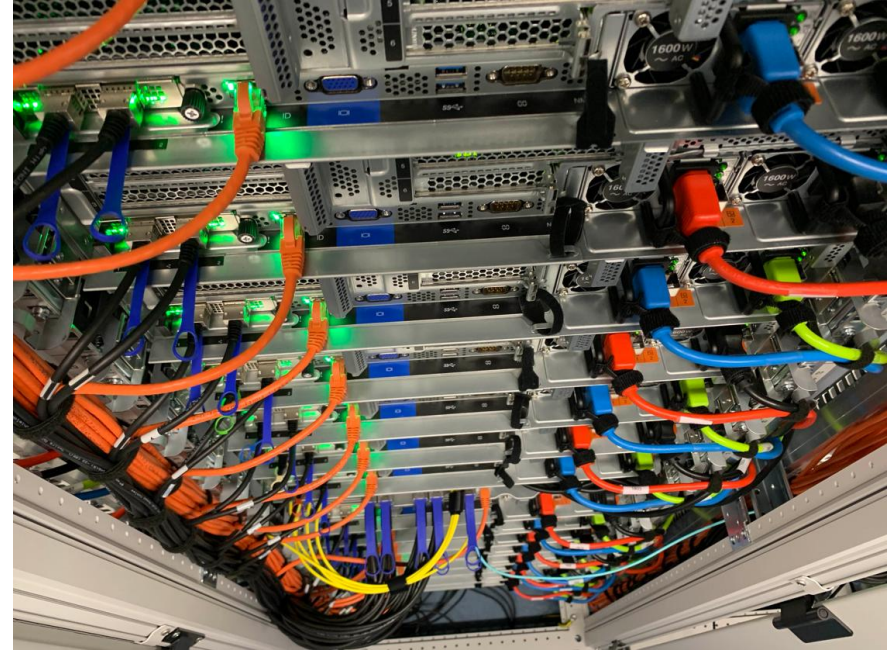
Image: Cluster ‘Lotenfeest’ at the Nikhef NDPF, acquired March 2020. Lenovo SR655 with AMD EPYC 7702P 64-Core single-socket. Some with 4 L40s Nvidia GPUs
