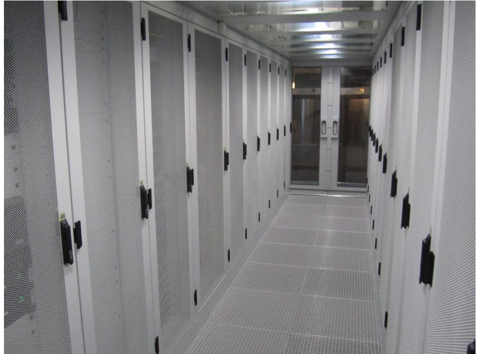
NikhefHousing: a cold aisle
