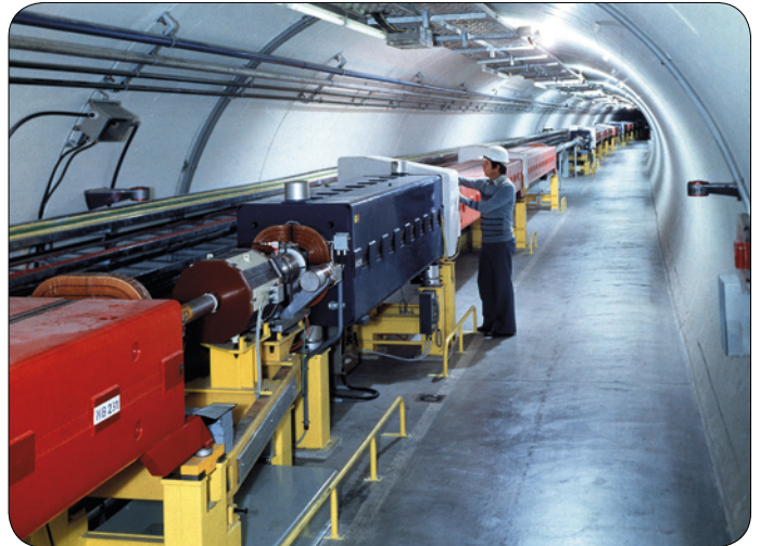
Figure 1. Last stage of preparation in the SPS tunnel at CERN (April 1976).
