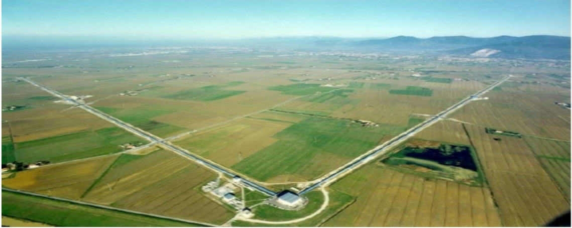
Figure 25: The French-Italian-Dutch Virgo detector is an interferometer with 3 km arm length. Together with the two LIGO detectors in the US it is poised to make a first gravitational wave detection in the next several years.
