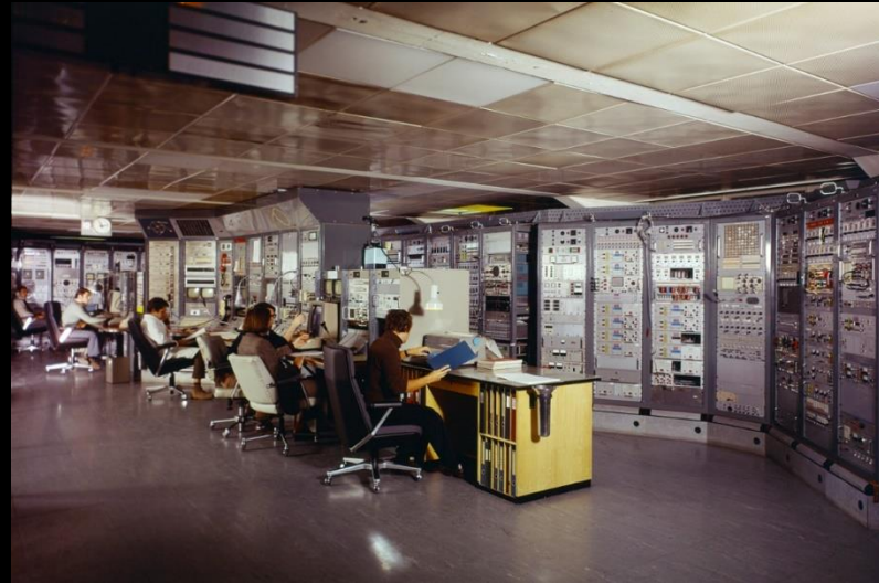
Image: PS control room at CERN
