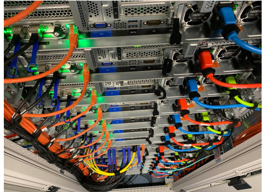
Image: Cluster ‘Lotenfeest’ at the Nikhef NDPF, acquired March 2020. Lenovo SR655 with AMD EPYC 7702P 64-Core single-socket
