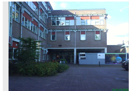
Entrance to NIKHEF, Kruislaan 409, just left of the grey metallic building (which contains the bike shed and a no-break UPS and diesel generator)
