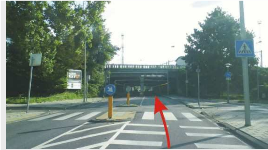
View on the Kruislaan, on your way to the Science Park from the Middenweg. The tunnel (about 150 metres long) crosses under the railway shunting yard. NIKHEF and the Science Park are beyond.
